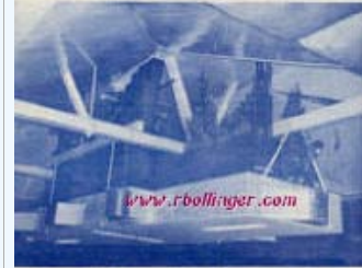
The organ loft, showing the largest organ in the United States, raised above the center of the huge rink floor. The new Oaks Rink Organ has 1,242 pipes, 2,525 magnets, 4,700 pouches and 500,000 feet of wire.
