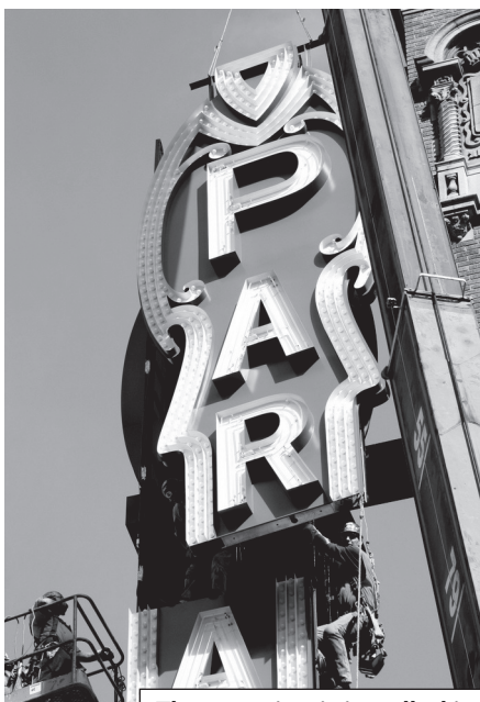
The new sign is installed in large sections, each 15 feet tall!
