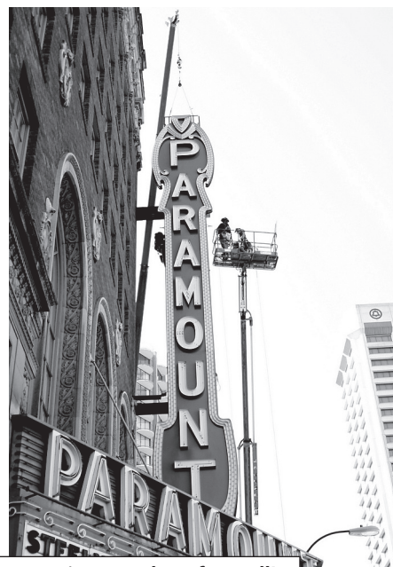
The new sign is installed in large sections, each 15 feet tall!
