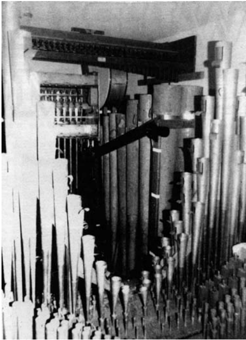
Excellent view of the Bauscher chamber areas is possible by means of employing the swing-out swell shade frame that rolls out into the studio. Chamber floor is several feet below studio floor level.
