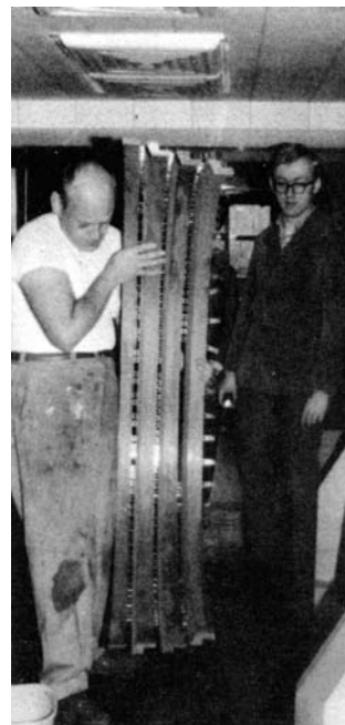
Lee Bauscher holds the new three-tiered stop rail assembly to show fellow organ buff, Ed Zollman, how it will replace the present stop rails on the Wurlitzer console.
